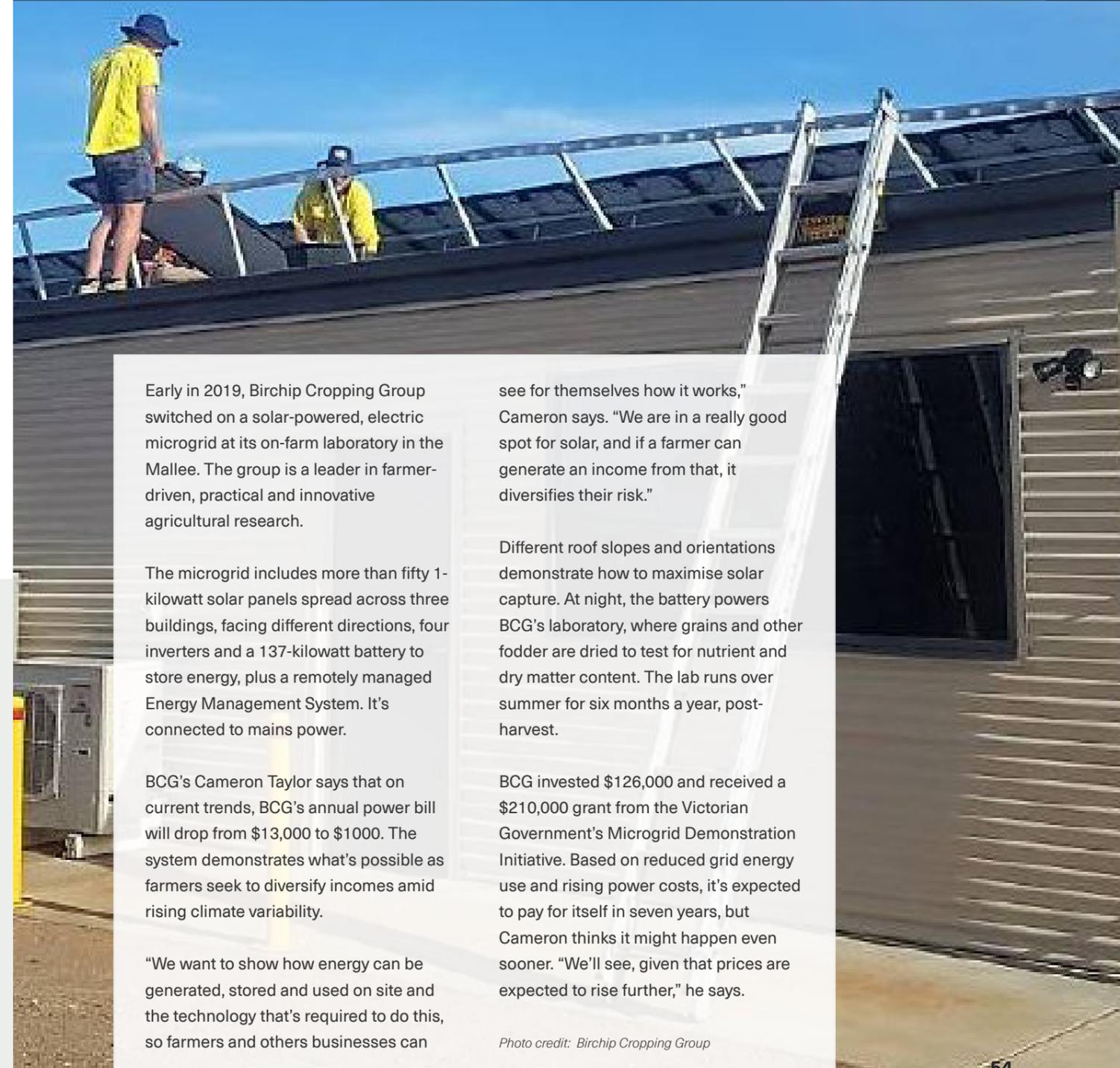
Early in 2019, Birchip Cropping Group switched on a solar-powered, electric microgrid at its on-farm laboratory in the Mallee. The group is a leader in farmer-driven, practical and innovative agricultural research.
